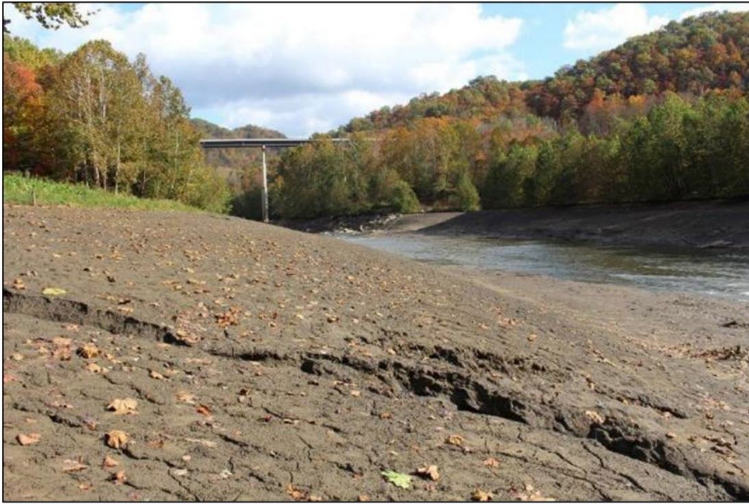
Figure 25. This is the section of the lake between the R.D. Bailey Lake Boat Launch and the Co Hwy 9/1 bridge. This section is inundated at the summer pool elevation of 1035' but is free-flowing during winter pool. This area is shown as purple on Figure 23.
